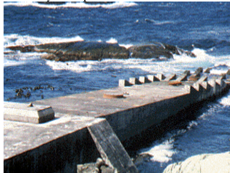
Figure 1 - Karmoy Immersed tubes. The fine pores in the silica fume concrete became totally filled by the seawater hydration products.
