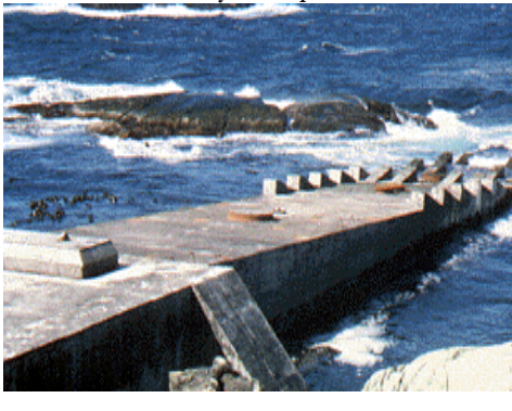
Figure 1 - Karmoy Immersed tubes. The fine pores in the silica fume concrete became totally filled by the seawater hydration products.
