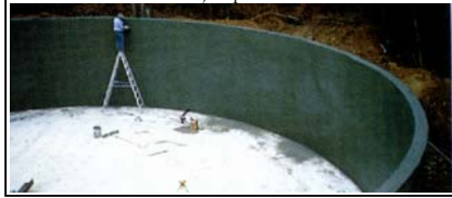
Fig 1b - Water tanks 20m diameter and 5m tall have been constructed in one day with silica fume shotcrete. An internal shutter about 3m long and full height is moved like a horizontal jump form.
