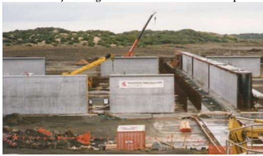
Fig 6 – Silica fume SRC was used for Blackrock sewage works. With the facility only 500 metres from Bass Strait, all concrete used was subject to high levels of chlorides as well as sulphates
